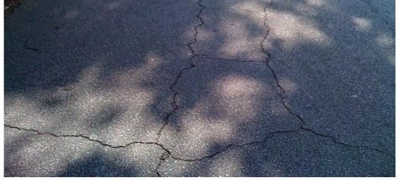
Fig. Block Cracking
