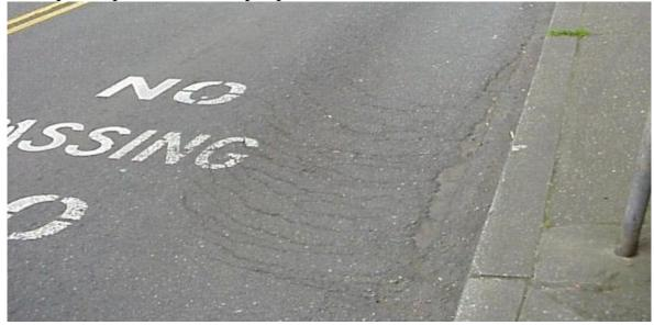
Fig. Slippage Cracks
