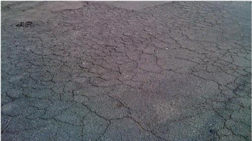
Fig. Alligator Cracking
