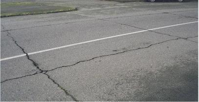
Fig. Joint Reflection Cracks
